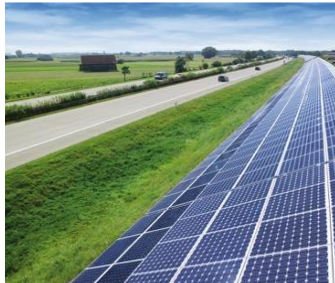
Solar – Installation to Maintenance
